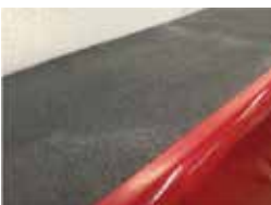
Anti-slip runway traction surface
